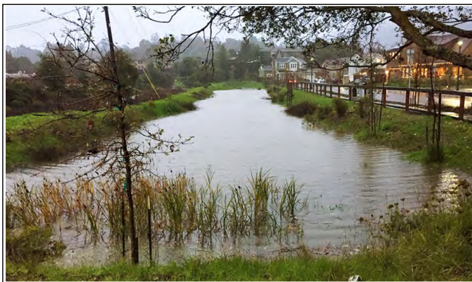
The swale, about 550 feet long, is located at the east end of the Rose Lane development, parallel to Larkspur Creek. The swale filled after a big December storm, and is seen from Doherty Drive. Photo by Sandy Guldman
