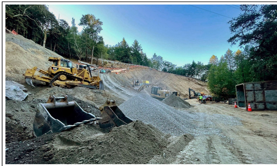
Major excavation is required to accommodate two new water tanks downhill from Sky Oaks Road. Photo by Gary Leo
